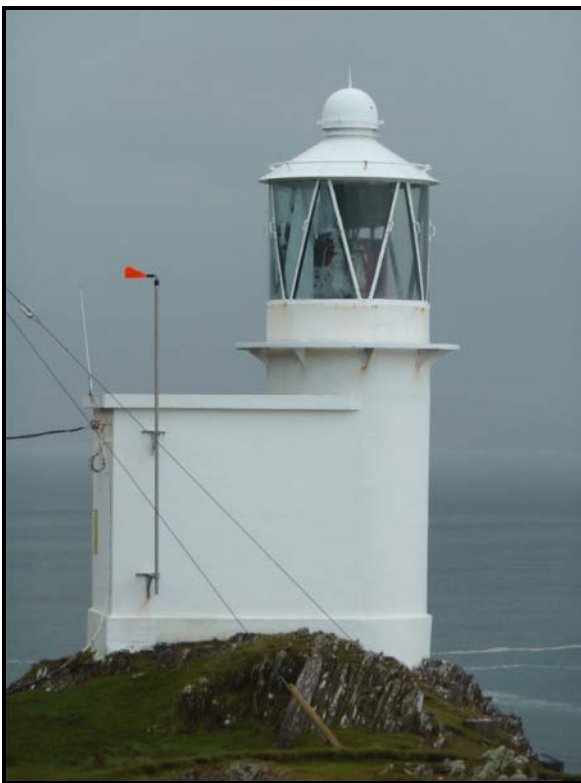
Achillbeg Lighthouse Ireland, Co. Mayo showing main and secondary optic.
