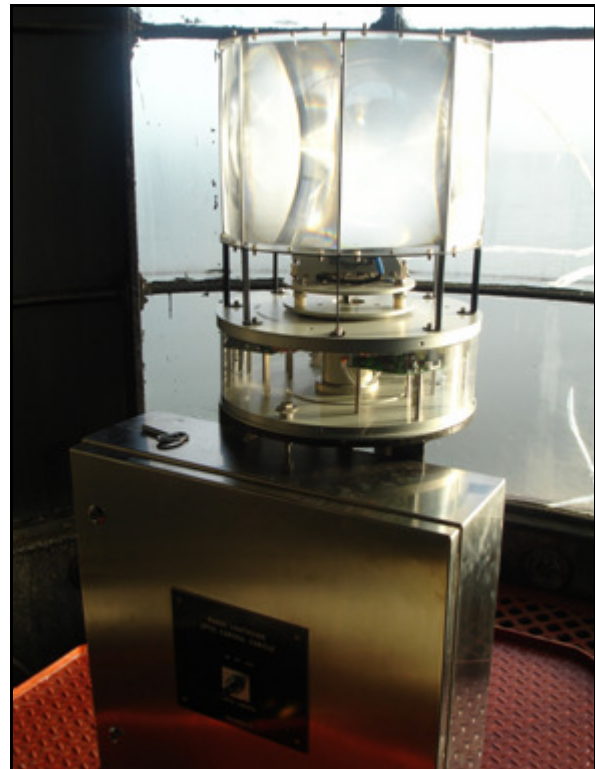
8 Panel - PRL400 pedestal and controls: Roker
