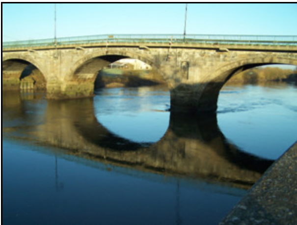
Trent Bridge looking down river showing the old lanterns marking of the centre span taken from East.
