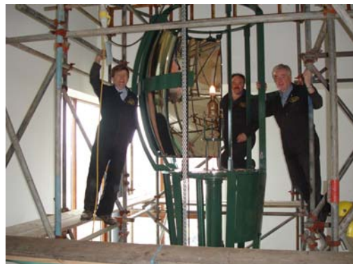
Optic installed in Museum
