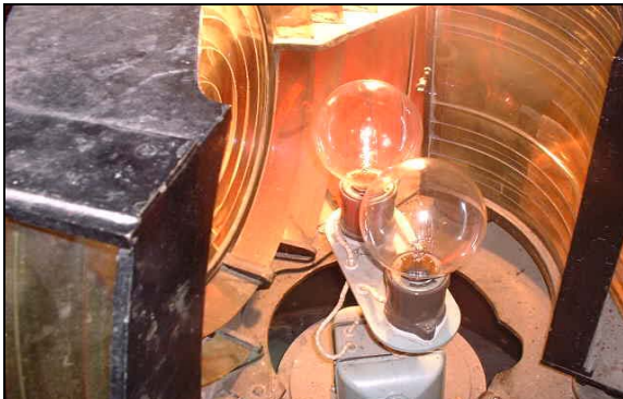
3 rd order lower Drum lens section with LC15.
