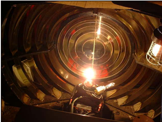
PA2 lampchanger installed in lower lens with 70 watt Cdmt lamp lit in position no 1.
